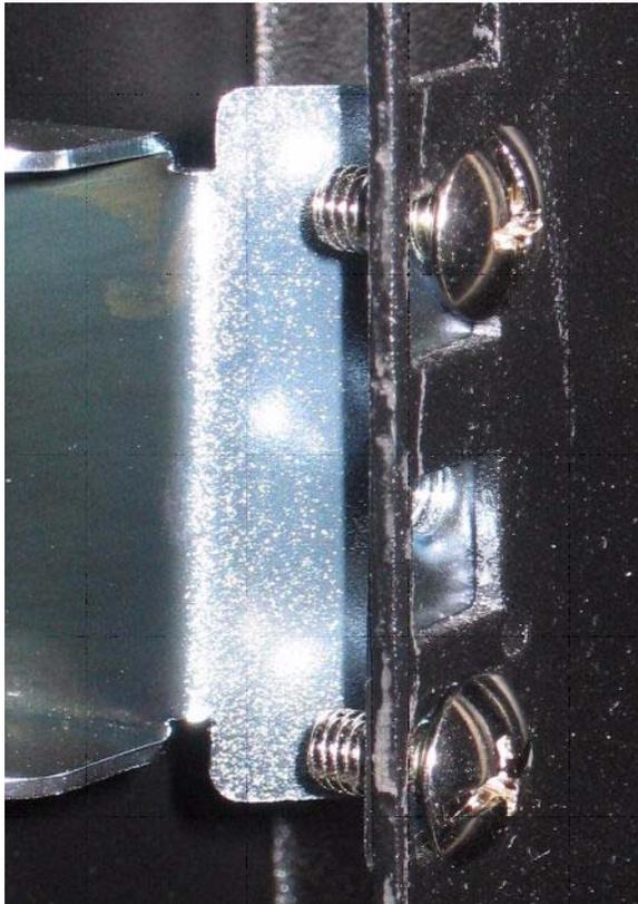
*Figure A.3 Mounting bracket attached to rack post*
